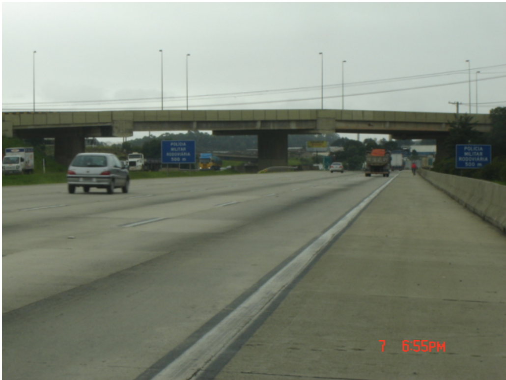
Passagem superior – km 13,0
