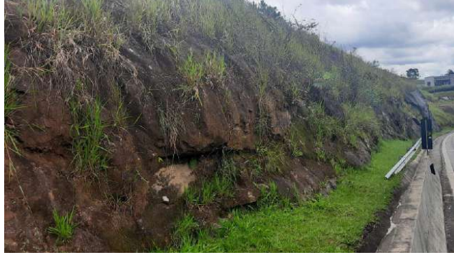
Figura 12: Talude 01 - Solo residual.
